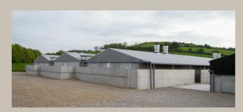
Animal welfare and comfort are key priorities when building or refurbishing your farm building. Pig buildings need to be able to withstand the aggressive and corrosive environments created by the pigs. Fibre cement is the ideal solution for this as it will not corrode in the ammonia rich environment.
