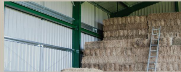
The crops need to be kept cool and dry. Euronit sheets can help with this as they not only have good thermal performance to keep the heat from outside at bay, they also retain moisture to reduce the chance of any dripping on the crops.
