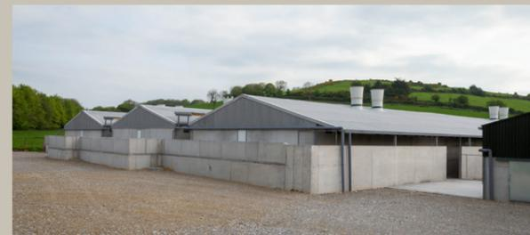
Animal welfare and comfort are key priorities when building or refurbishing your farm building. Pig buildings need to be able to withstand the aggressive and corrosive environments created by the pigs. Fibre cement is the ideal solution for this as it will not corrode in the ammonia rich environment.
